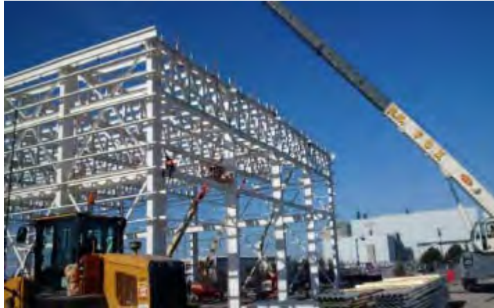
Erection of structural steel
