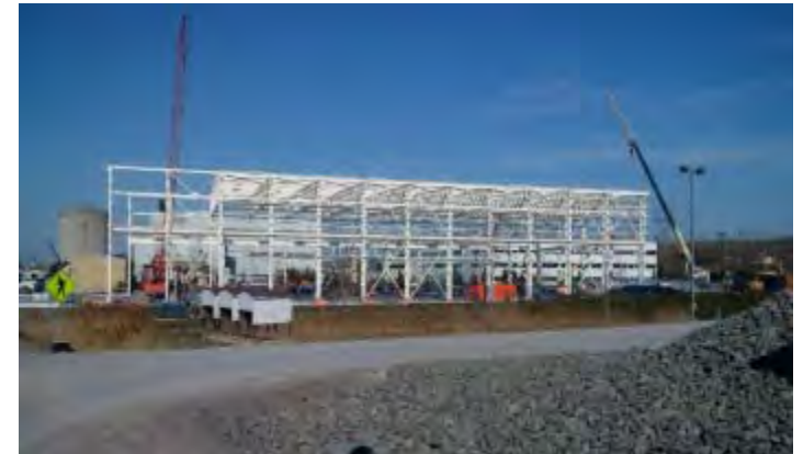
Erection of structural steel
